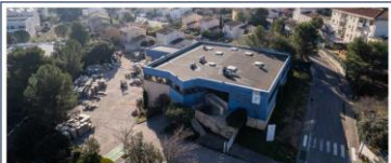
TRANS DISTRIBUTION à Aix-en-Provence PAAP 1 250 m 2 - Location – 2 nd main
